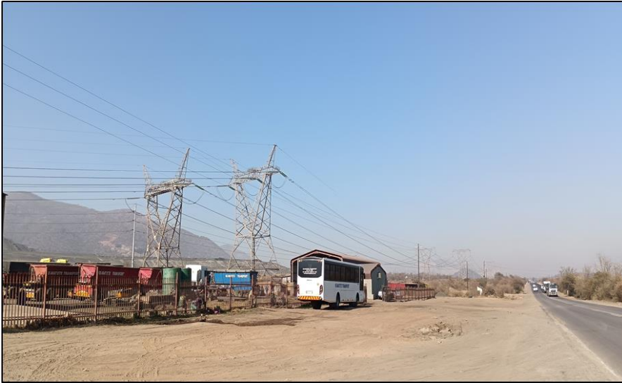
Figure 3-11: Photo taken towards southwest along the R555 road indicating high voltage powerlines in the area.
