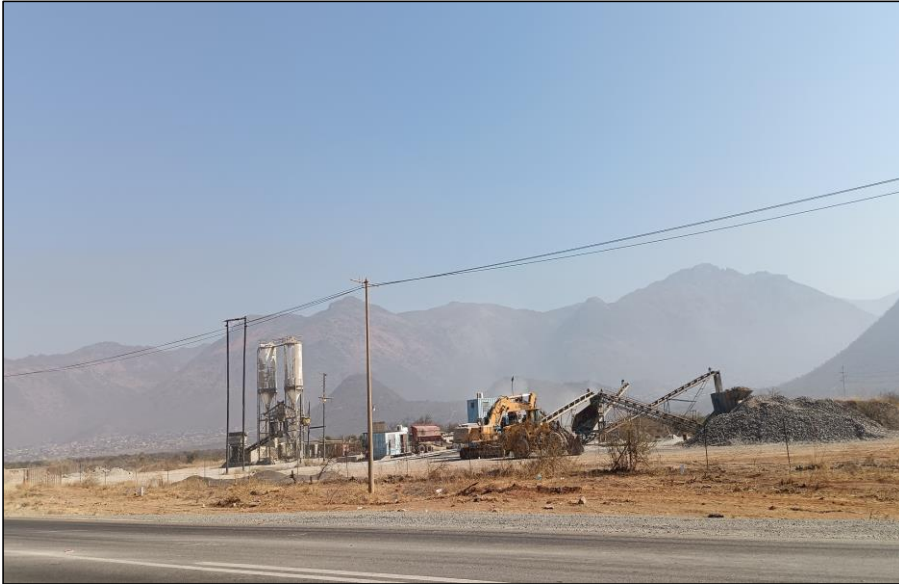
Figure 3-15: Photo taken to the northwest towards the Project site indicating degradation due to mining developments.
